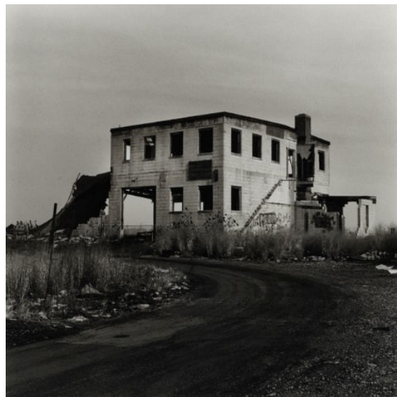
Abandoned Building. Caven Point. N.J. 1984
